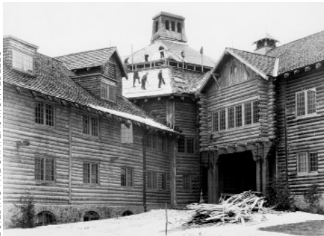
BUILDING THE CHATEAU MONTEBELLO
